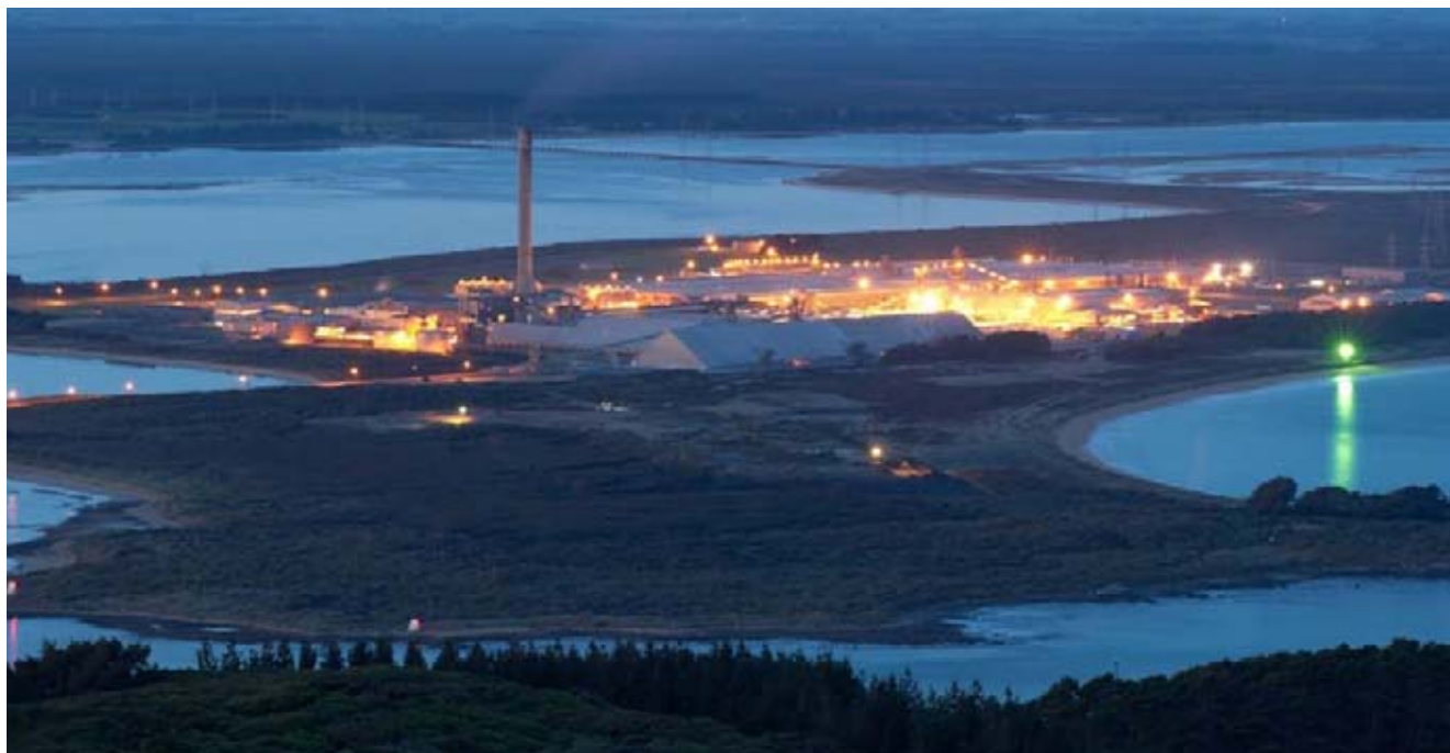
Night view of smelter.
